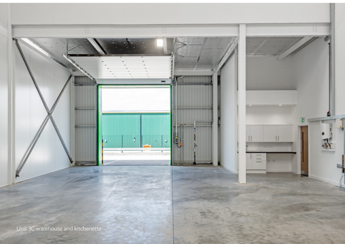
Unit 3A warehouse
