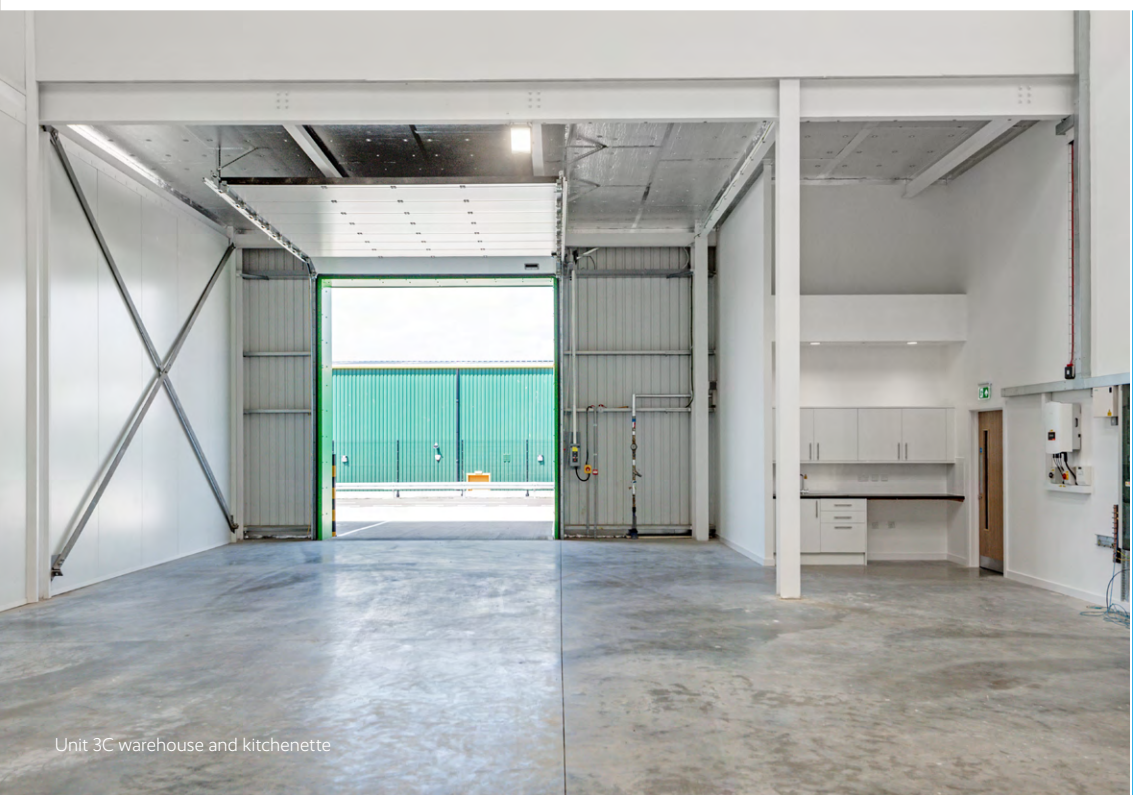
Unit 3A warehouse
